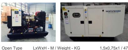
LxWxH - M / Weight - KG Canopied Type LxWxH - M / Weight - KG 1,5x0,75x1 / 475 1,75x1x1,2 / 625
